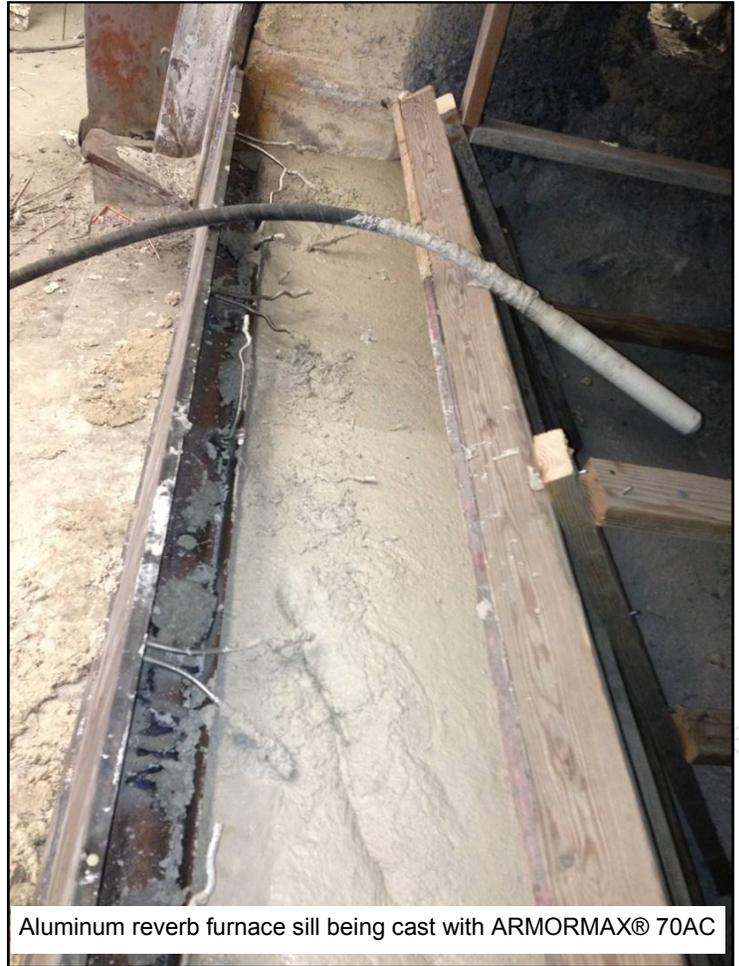
Aluminum reverb furnace sill being cast with ARMORMAX® 70AC
