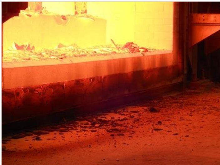
ARMORMAX® sill after 1 month in service
