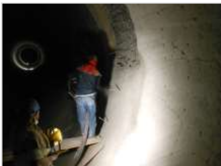
Shotcreting de TUFFCRETE 90
