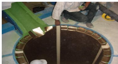
Figure 8 - Mica Sheet Installation
