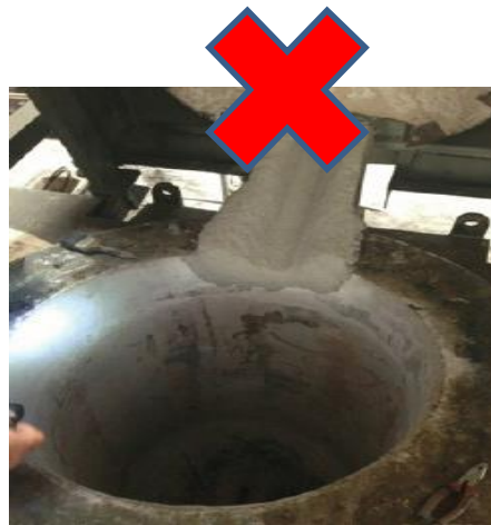
Figure 6 - Installed Spout with A 7055
