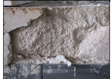
Spalling and cracking with competitive castable
