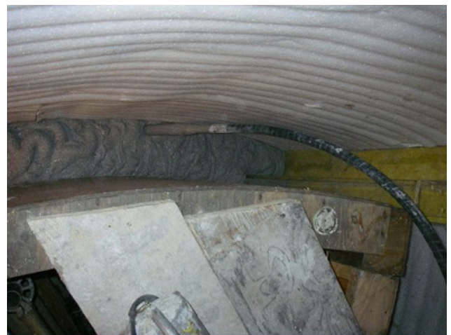
Pouring of combustion chamber wall
