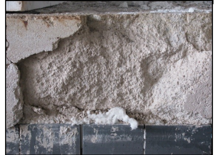
Spalling and cracking with competitive castable
