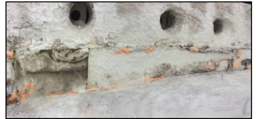
Top charge furnace before QUICK-FIRE® installation
