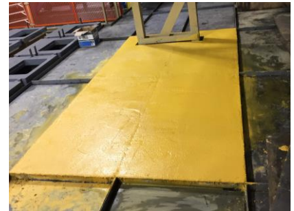
Installation of yellow TUFFLOOR section
