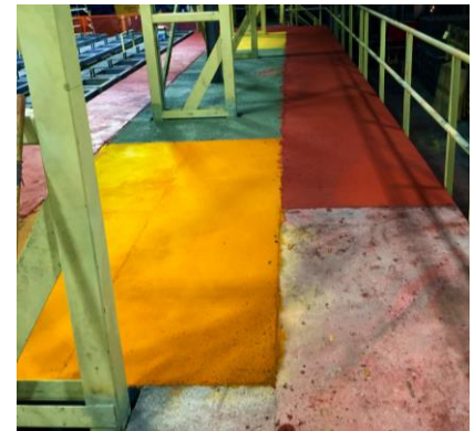
Completed TUFFLOOR flooring sections
