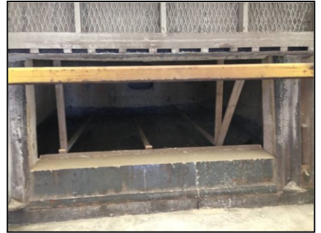
Installed sill
