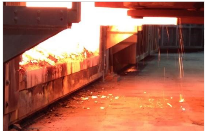
ARMORMAX® sill after 18 months in service
